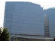
Guangzhou FA Center MITSUBISHI ELECTRIC AUTOMATION (CHINA)LTD.
