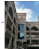
Mexico Monterrey FA Center Monterrey Office, Mitsubishi Electric Automation, Inc.
